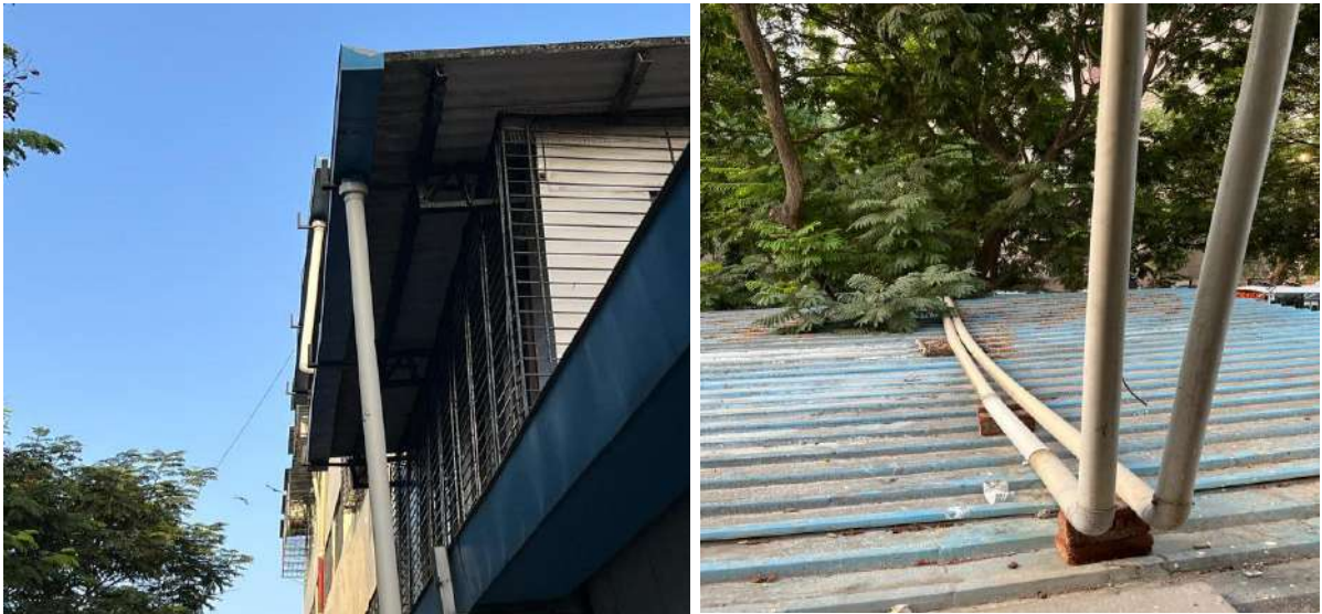
Disposal Pipes Diverting Roof Water down to Garden Area
